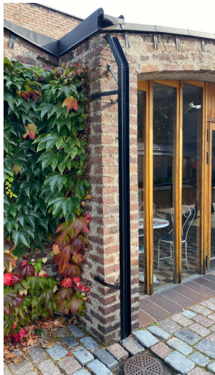
Gutter and drainpipe design
