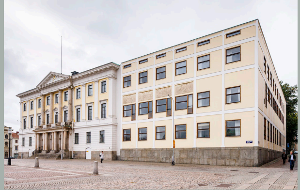
Exterior photo Göteborg Law Courts Annex ©2023 Gareth Gardner. All rights reserved
