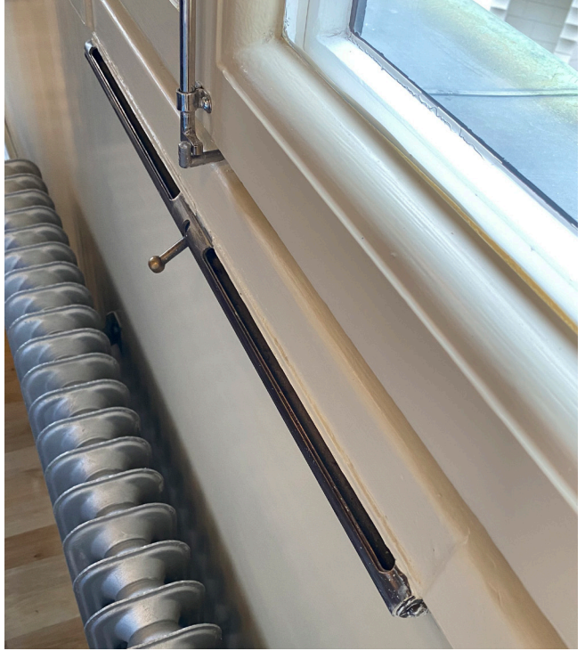
Marginalen Bank ventilation detail
