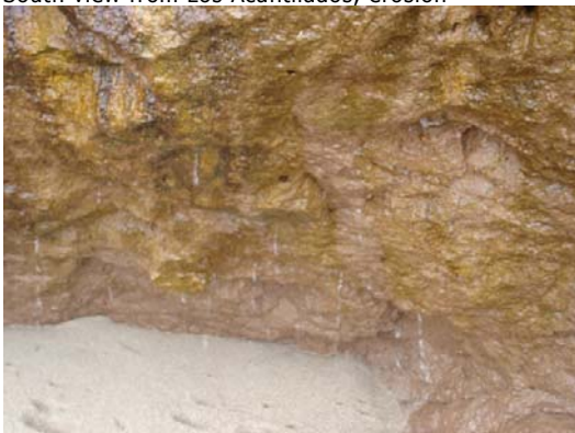
Leaking groundwater trough the cliffs
