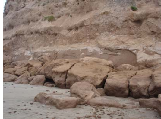
Big parts of the cliff fall off, clearly visible how the rock easily break in two.
