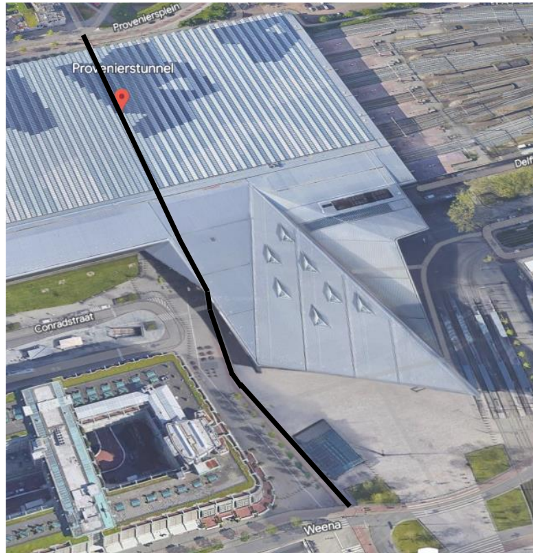
Figure 2, Birds-eye view on the Provenierstunnel at Rotterdam central station. Adapted from (Google, n.d.)
