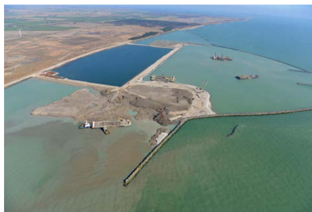
Figure 2.19: Dredging activity in the Fehmarnbelt, Germany (“Fehmarnbelt Fixed Link Dredging and Reclamation, 2021” by Royal Van Oord is licenced under CC BY-NC-SA 4.0).
