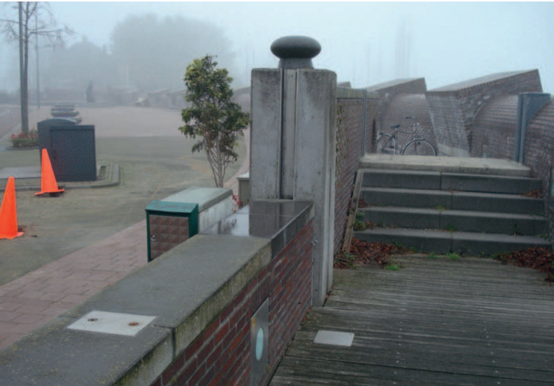
Figure 4. MFFD Kampen, touristic walkway integrated in flood defense structure (photo courtesy Mark Voorend)
