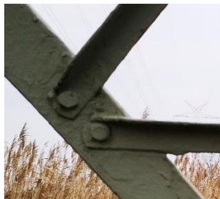
Figure 119 Single leg bolted connection
