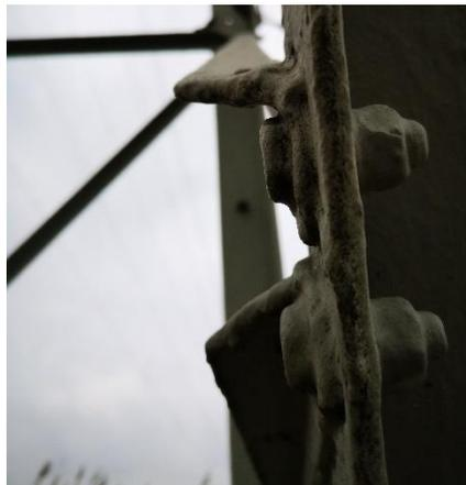
Figure 133 Unsymmetric bolted connection in the in-situ structure
