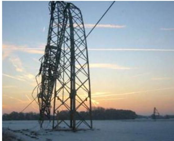
*Figure 1 Collapse of the lattice tower [1]*
