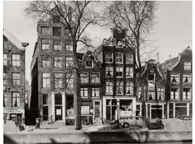
Figure 20: Inclination of the building (Stadsarchief Amsterdam, 1955)
