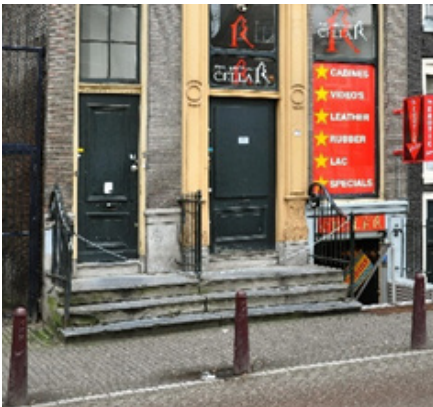
Figure 31: Elevated entrance (Amsterdam Stadsarchief, 2009)
