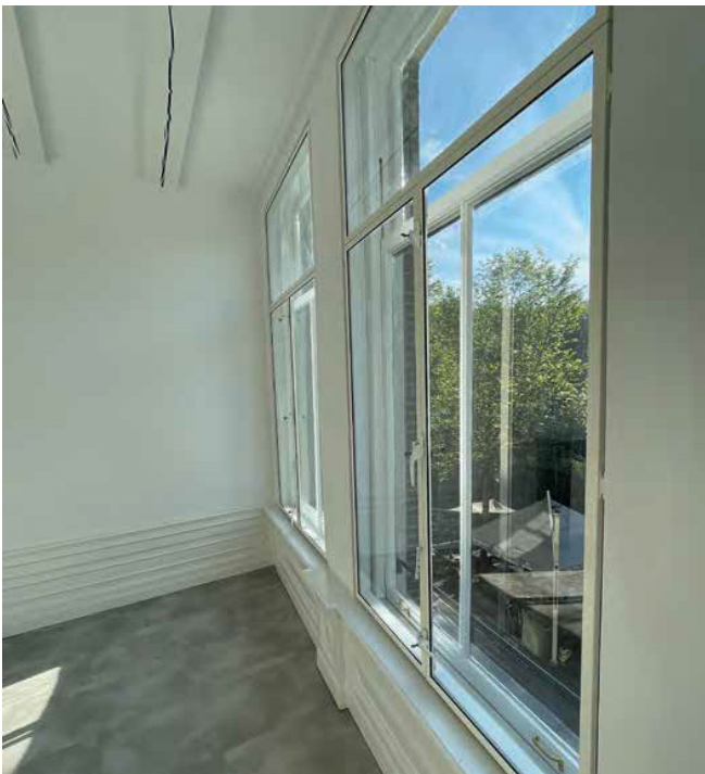
Figure 27: Secondary glazing incorporating vacuum glass (Van Cappelleveen, 2022)
