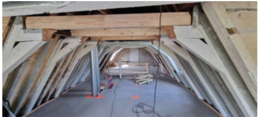
Figure 32: beams were sawn through providing an additional height of 20 centimeters (Veldt, 2022)
