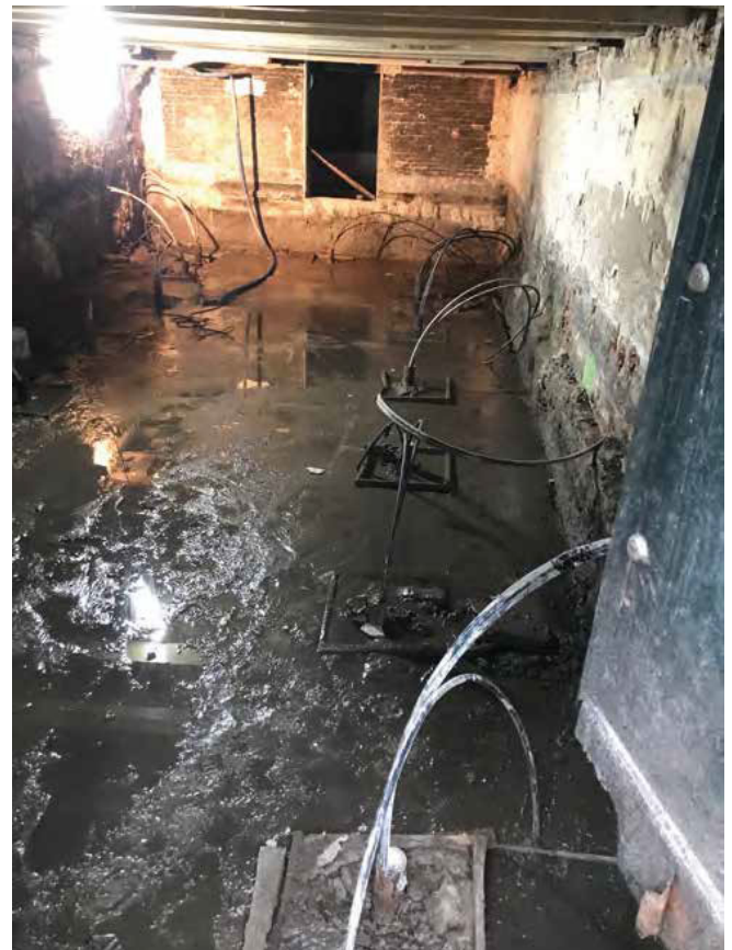
Figure 23: Nineteen Green Poles were installed in the new basement (Veldt, 2022)
