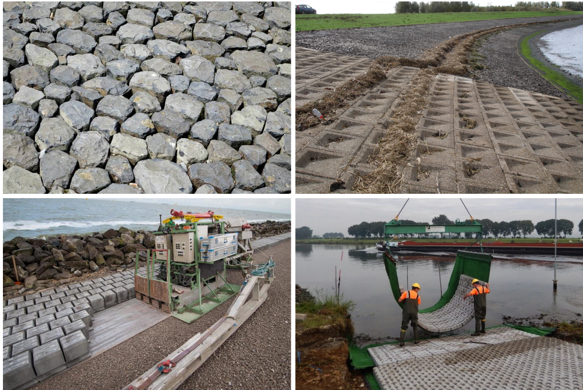
Figure 2.3: Different types of pattern-placed revetments: top left: basalt columns (Stenen zoeken.nl, 2020), top-right: Haringman blocks (DeltaExpertise, 2020), bottom-left: Interlocking Verkalit elements (LBN Beton, 2020), bottom-right: RonaTon block mats (Altena Infra-materialen, 2019)
