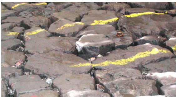
Figure 3.3: Partially uplifted elements (left, Klein Breteler and Eysink, 2005) causes loss of clamping (right)
