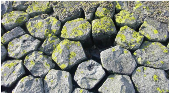
Figure 3.2: Missing elements (left, Waterschapshuis, 2019) causes a loss of clamping (right)
