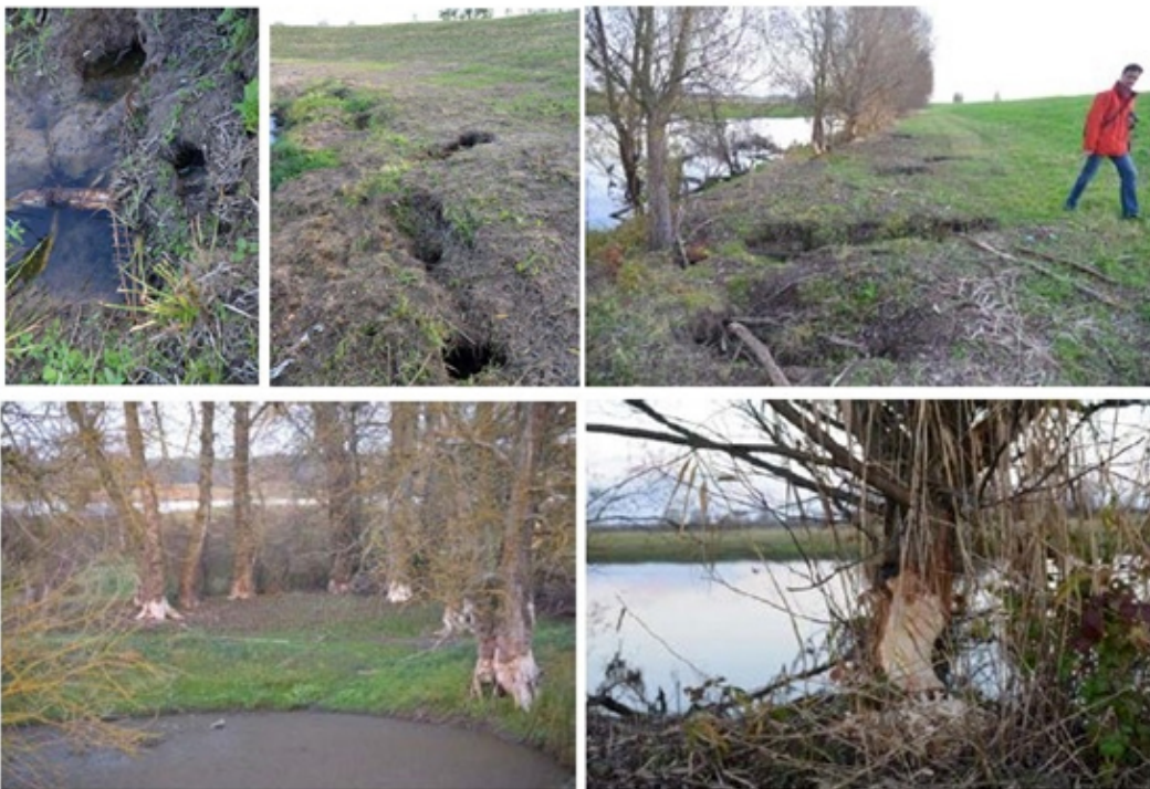
Figure 3. Effects of beavers in floodway encroachment zones along the Odra river in Sophienthal (Germany)
