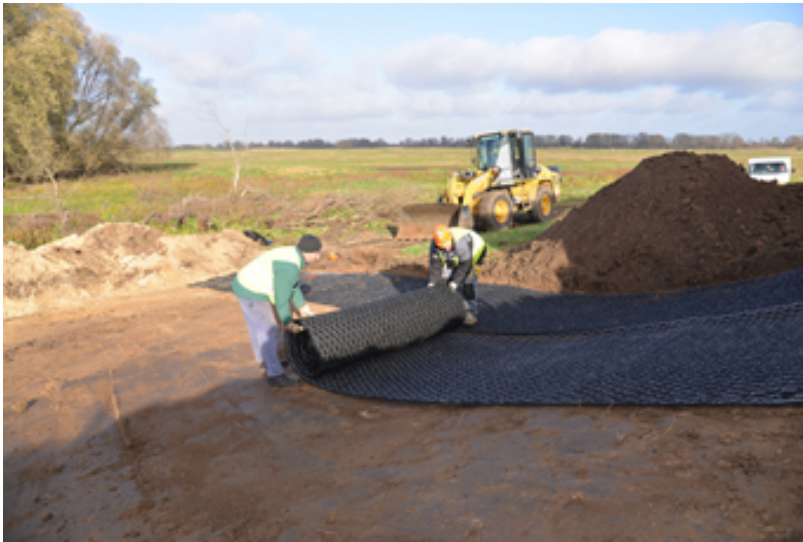
Figure 4. Installation of beaver netting
