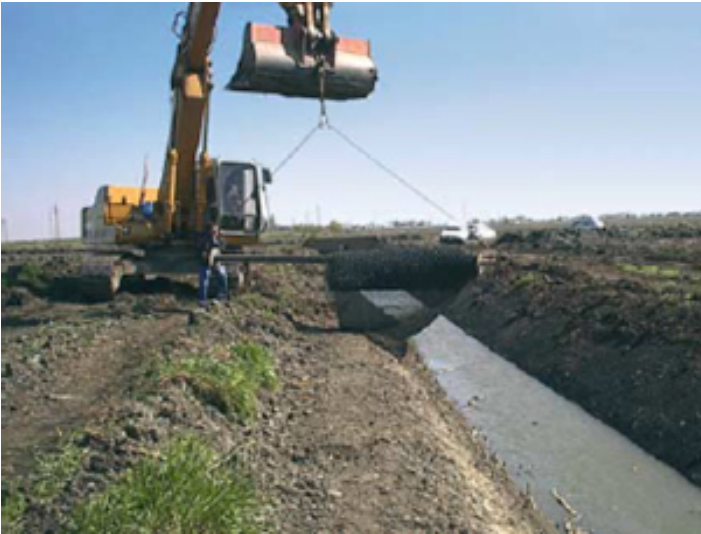
Figure 5. Installation of beaver netting along Zabarelle Canal
