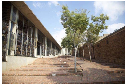
3.3.9 The African steps with at the left the Constitutional Court and at the right an old prison wall.
