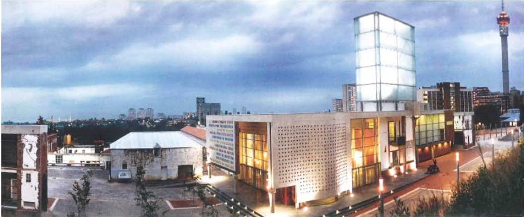
3.3.11 The building volume of the foyer and court chamber seen from Constitutional Square.
