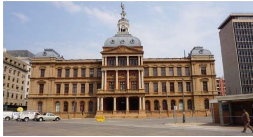
2.2.8 The front facade of the Raadzaal .
