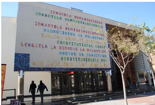
3.3.16 The light translucent structures above the old staircases.
