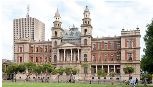
2.3.5 Final realized front facade with three floors.
