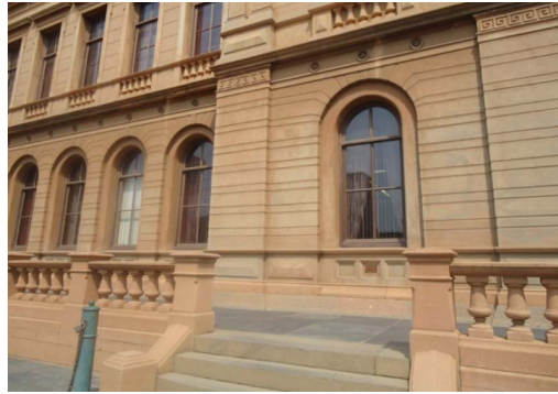
2.2.12 Facade of the Raadzaal . Notice the ciment-fondu balusters and plastered ‘sand stone’ walls.
