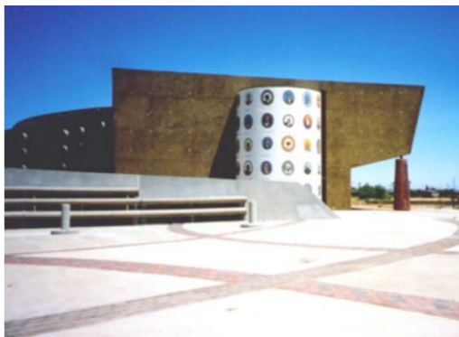
3.2.15 The facade of the Members of Parliament Building facing Peoples Square.
