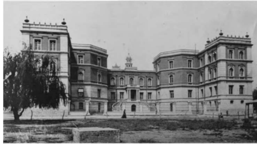
2.3.3 Back facade of the Paleis van Justitie .
