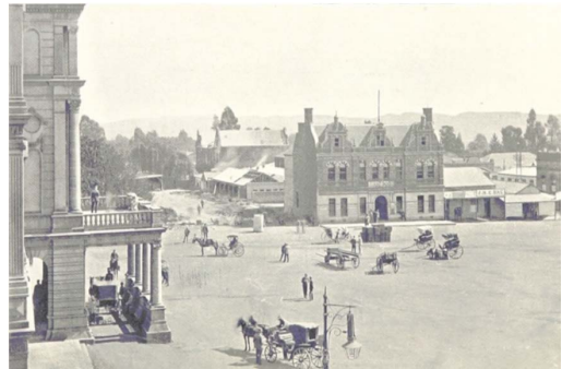
2.2.18 Paul Kruger leaving the Raadzaal in 1899. This shows the low threshold to the Raadzaal and the practical integration of the porte-cochère that creates both a dry entrance and a balcony on top from where the states man could speak to the public.
