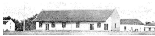
2.2.1 the first Raadzaal building. A simple single storey building with mud walls, a thatched roof and a stoep .
