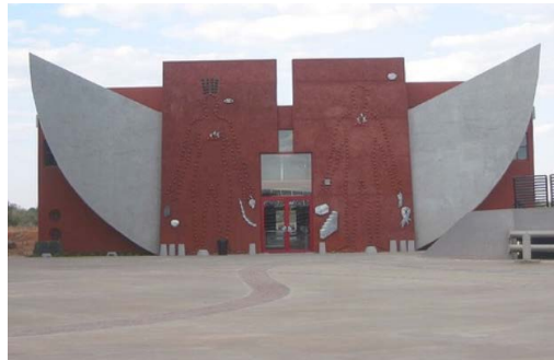
3.2.16 The facade of the Premiers Building.
