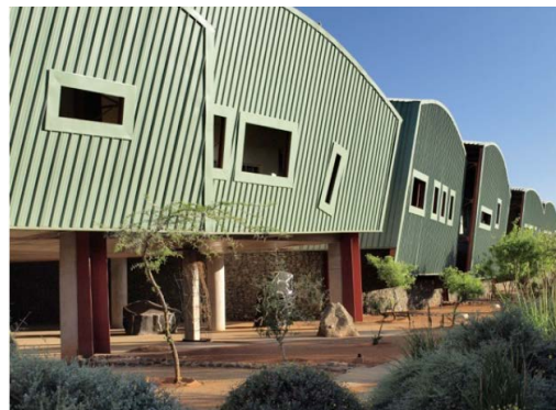
3.2.17 The administrative wing with its modernist light architecture.
