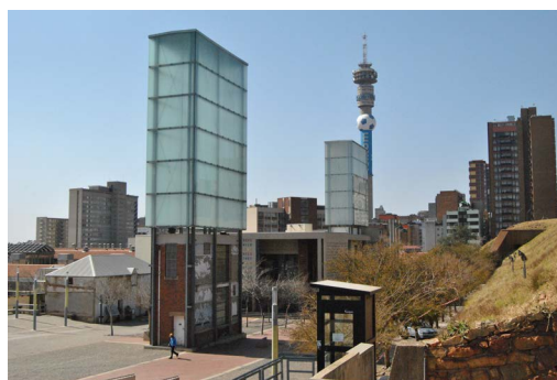
3.3.10 The light translucent structures above the old staircases.
