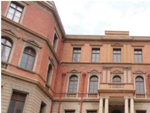
2.3.6 The sweeping stair at the north facade leading to the entrance for the judges.
