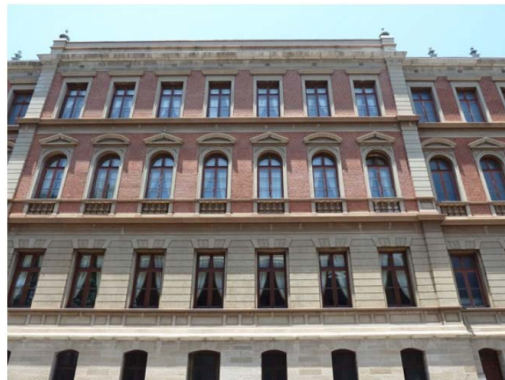
2.3.7 The western facade. Note the appliance of half round and triangle pediments above the windows on the second floor.
