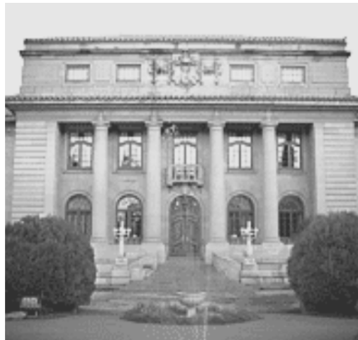
3.3.1 Court building of the Appellate Division in Bloemfontein.
