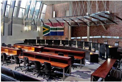
3.3.15 The reused brick of the prison on the wall behind the Judges benches.
