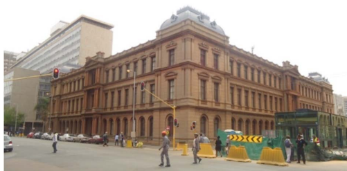
2.2.9 The north and east facade of the Raadzaal . Notice the similarities.
