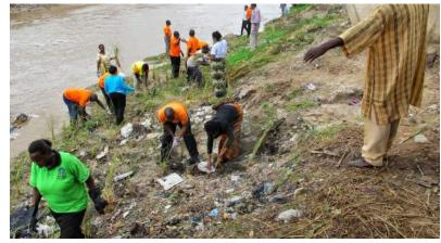
Figure 5 Some of Ilala Municipal Employees busy with vetiver grass planting preparations along Msimbazi river in Dar es Salaam to curb soil erosion and rehabilitate the environment 2015
