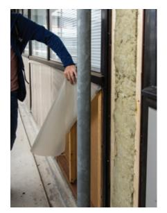
Figure 16 Wooden facade under thermal renovation (2016). Additional layers of mineral wool inserted for insulation.
