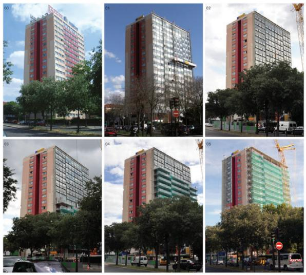
Figure 33 Process of new facade construction. Using this method, inhabitants did not have to leave their flats for the construction time.
