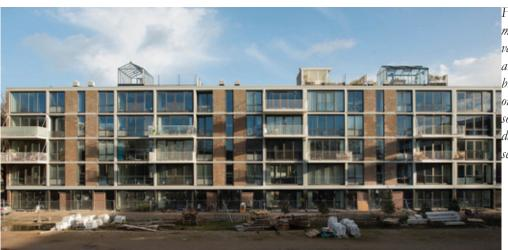
Figure 48 Facade after transformation: using similar materials, variation in form of balconies and roof terrace is introduced, breaking monotony of the previous design.
