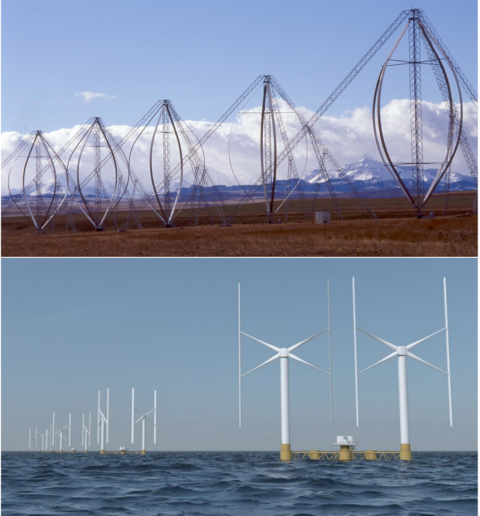
Figure 1.2: Upper: Adecon AL-38 turbines in Pincher Creek, Alberta. Photo by Jos Beurskens (Möllerström et al., 2019). Lower: The NENUPHAR concept of floating VAWT with a double 2 \times 5 MW rotor concept.
