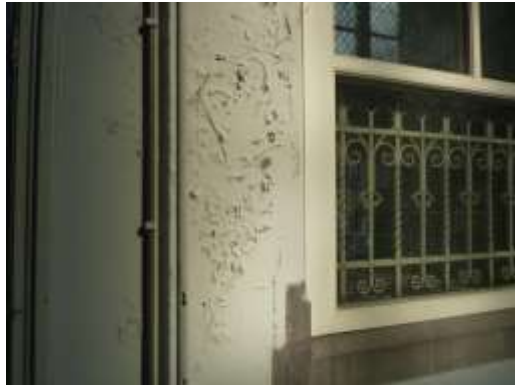
Efflorescence
