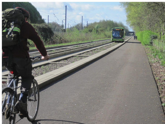
Fig. 1. The Cambridgeshire guided busway.
