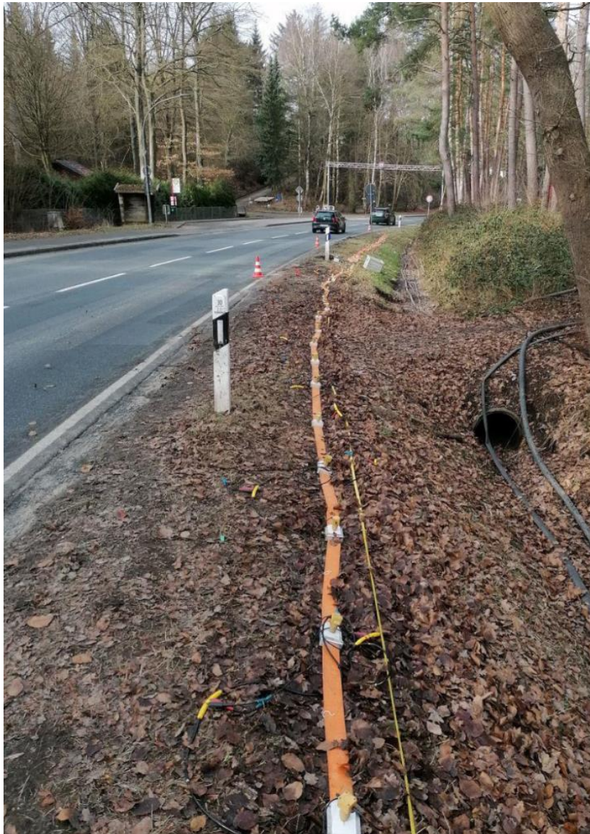
Figure 10 Land streamer on Emmetal road test profile
