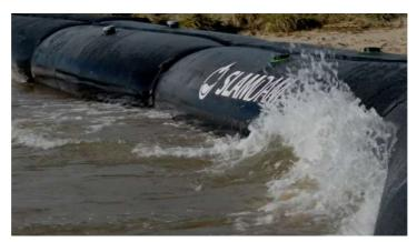
Figure 21: Slamdam: temporary flood defence that is filled with water (Slamdam (2019)).
