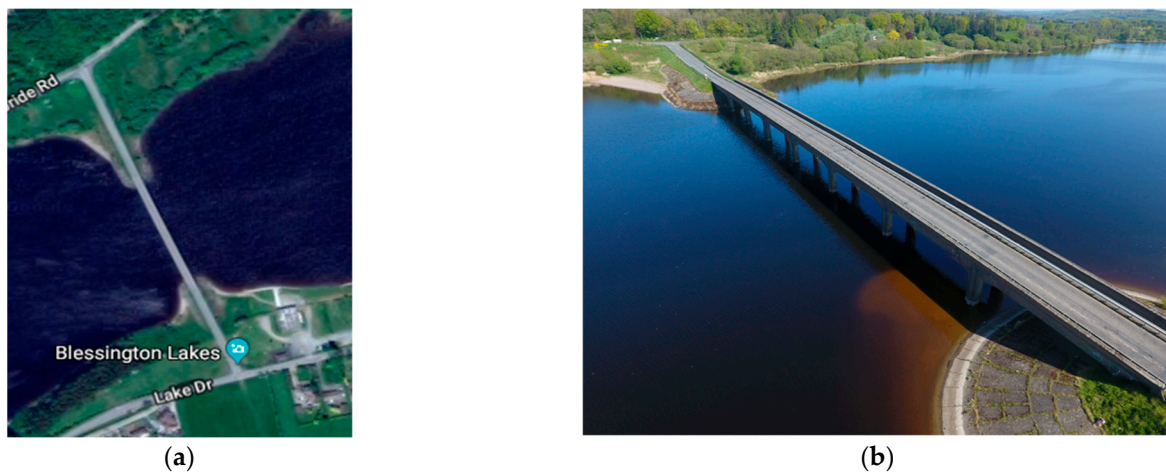
Figure 9. Blessington bridge and surrounding environs: (a) satellite image; (b) aerial image.
