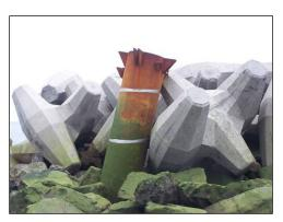
An inspection of the breakwater was carried out in June 2008 and confirmed the observed damage. Several Core-Loc units were found to have suffered damage during the structure's first winter. The number of breakages equates to approximately 1% of the total number [WAREING A.W. *et al.* 2009].
