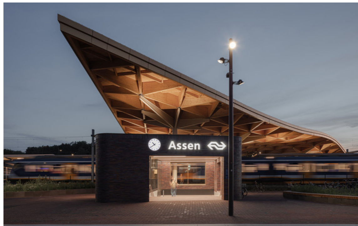
Assen Station, Netherlands Powerhouse Company + De Zwarte Hond
