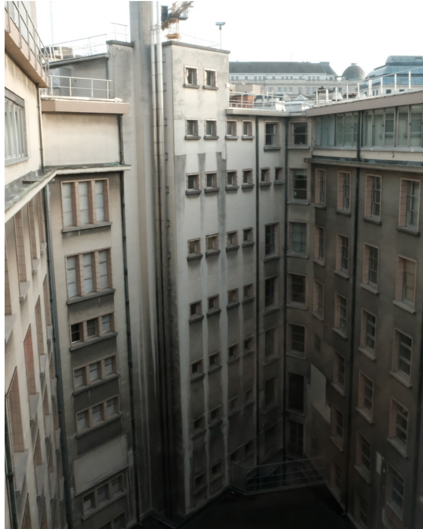
Internal (back) Facades of the National Bank of Belgium
