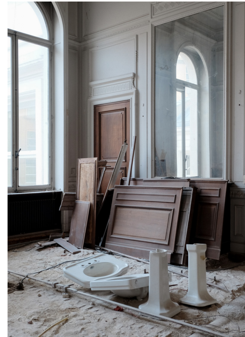
Governor's Palace National Bank of Belgium Photo: Bas Leemans
