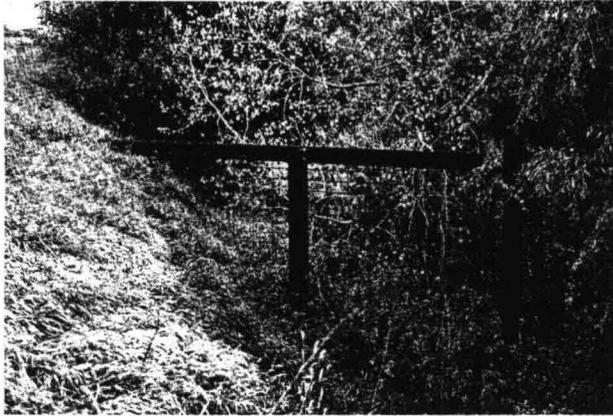
FIGURE 62. WIRE-MESH PERMEABLE SPUR ILLUSTRATING SPUR ROOT EXTENDING INTO CHANNELBANK.
