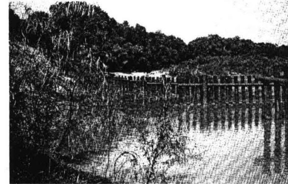
FIGURE 61. HENSON SPUR SHOWING OUTFLANKING.
