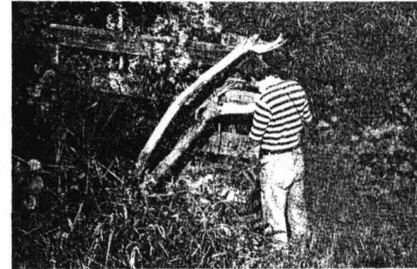
FIGURE 4. WOOD-FENCE SPUR; BATUPAN BOGUE, GRENADA, MISSISSIPPI.
