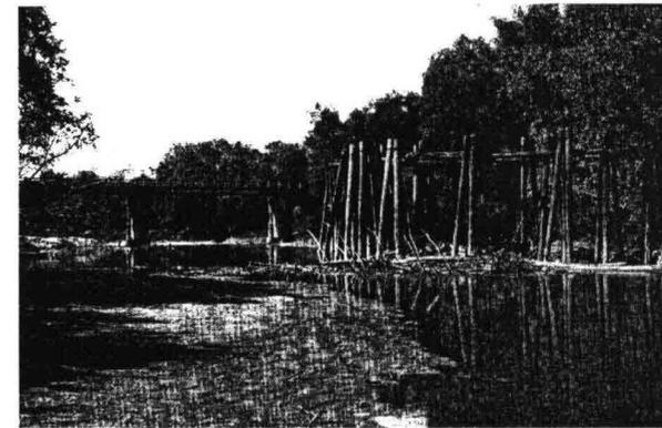
FIGURE 9. TIMBER PILE SPURS; BIG BLACK RIVER AT DURANT,
