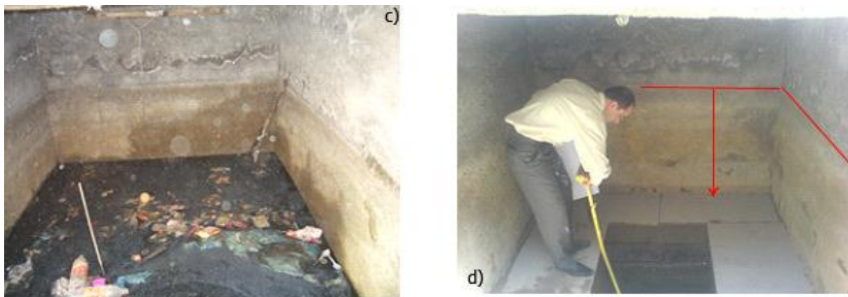
Figure 4: Qanat's outlet, before and a couple of days after revitalization.
