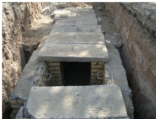
Figure 3: Typical cross section of the scheme, the concrete slabs (1-1) will be covered by aggregated soil.
