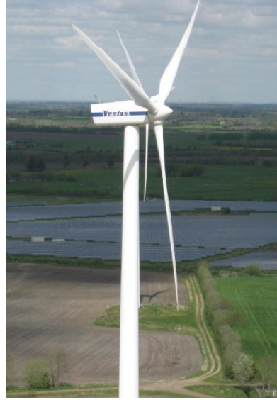
Fig. 3. The Vestas V66 wind turbine under measurement.
