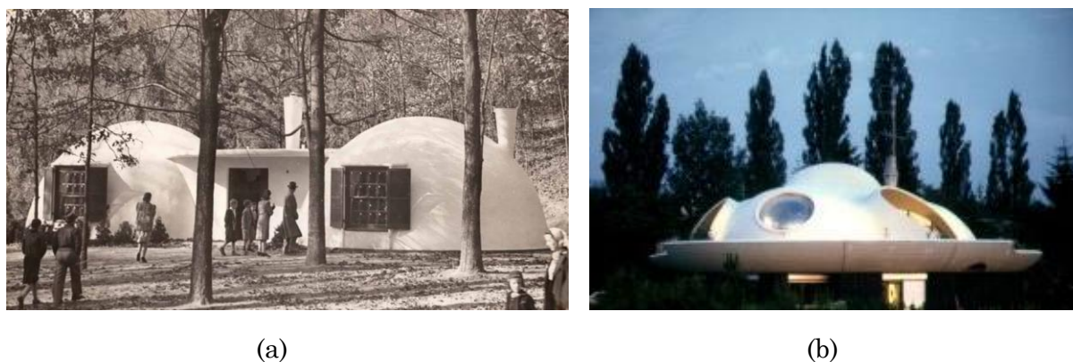
Figure 2.11 : Examples of shell structures achieved by spraying concrete onto a pneumatic formwork: (a) the Bubble Houses by Wallace Neff, Pasadena, California, U.S.A., 1946; (b) the Balz House by Heinz Isler, Stetten, Germany, 1980 (Balz, 2022) (photo credit: (a) Jeffrey Head).
