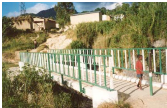
Figure 2.1 : An solid slab reinforced concrete pedestrian bridge in Malawi (Dennis, 2015)
