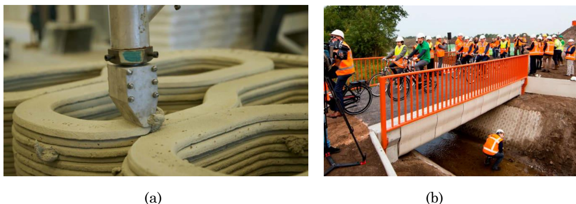
Figure 2.15 : (a) extruded 3D concrete printing; (b) the 3D printed cycling bridge by TU Eindhoven; (photo credit: (a) Houben/Van Mierlo architects; (b) Salet et al, 2018).
