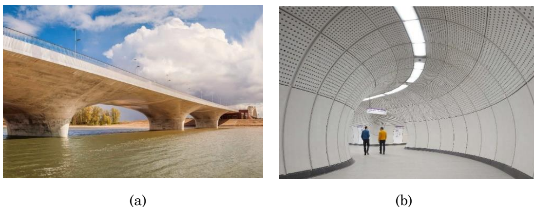
Figure 2.10 : (a) The Extended Waalbridge by ZJA, Nijmegen, The Netherlands, 2015; (b) The Elizabeth Line by Grimshaw, London, United Kingdom, 2019; (photo credit: (a) Raymond van der Hoogt; (b) Grimshaw).
