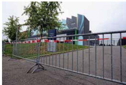
11. Current state of Kerkrade Campus. Built only a few year ago, the complex is now totally abandoned by all of its tenants, due to a combination of construction faults and too high prognoses for success of the school. Source: Trompetter (2013).
