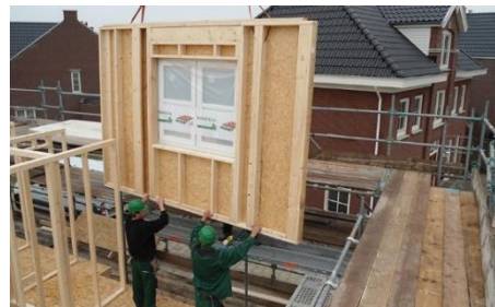
FIGURE 45: HSB WALL (DE KROON PREFAB, N.D.)
