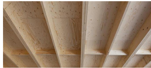
FIGURE 35: KERTO LVL FLOOR (METÄWOOD, N.D.)
