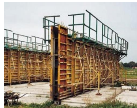
FIGURE 41: CAST IN SITU WALLS (BETONHUIS, N.D.-A)
