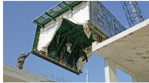
FIGURE 31: GIETBOUW (BETONHUIS, N.D.)
