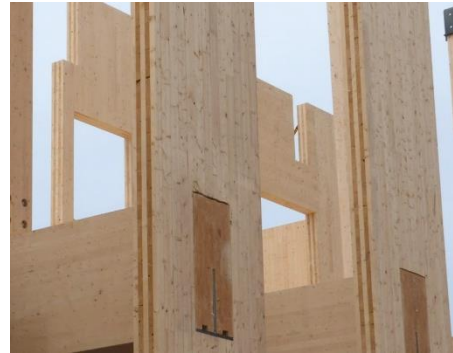
FIGURE 43: CLT WALL (ALTER, 2019)
