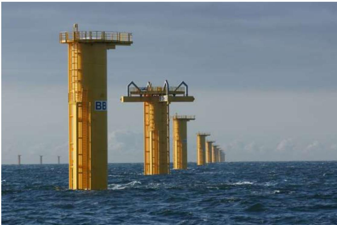
Figure 8: Installed offshore monopile wind turbine foundations with transition piece<sup>ii</sup>
