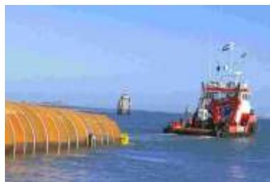
Figure 18: Towing monopile on the monopile and not the end-cap
