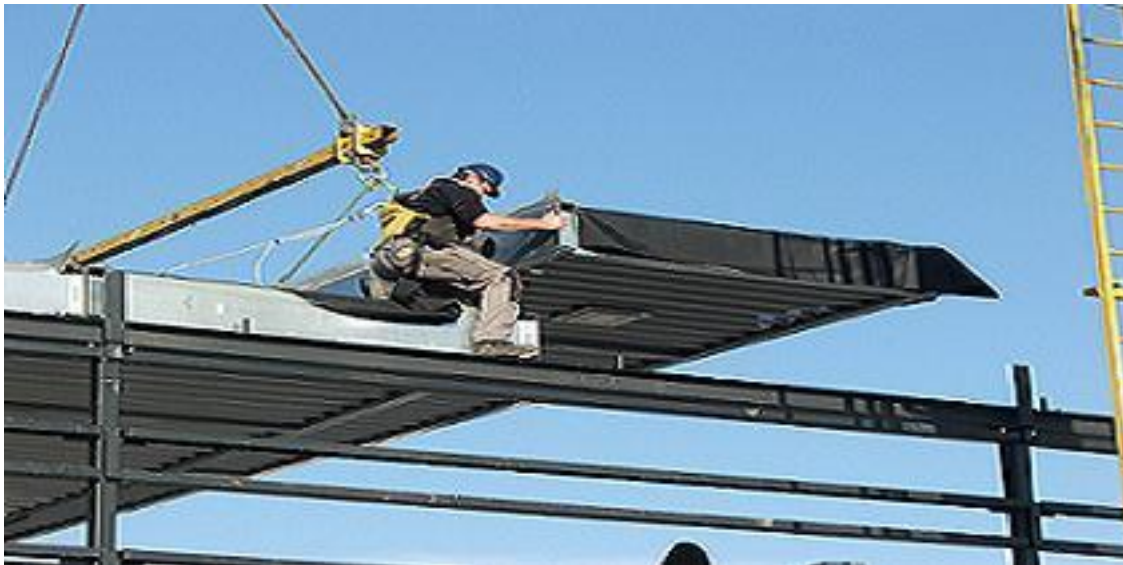
Figure 4.2, Steel-wood system from www.flex-frame.nl
