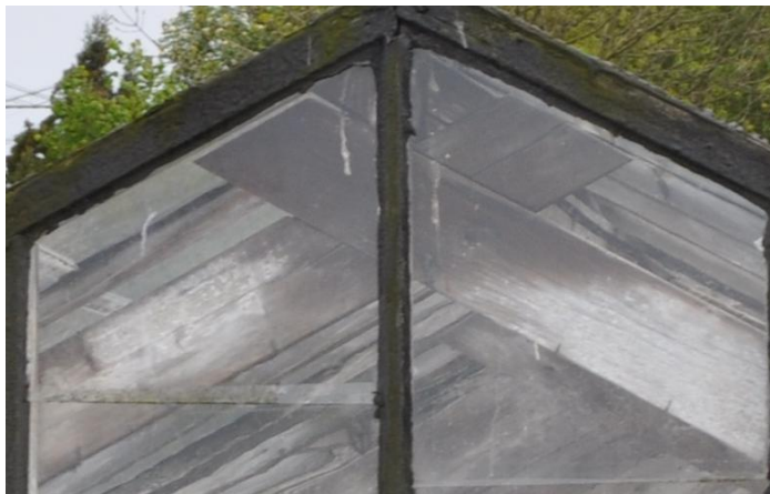
Figure 4.16, diagonal lap joint
