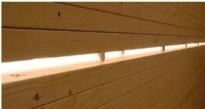
Figure 4.19, Wood pins to form a wall or floor, sources: Inholz.de , www.kaufmann-holzbau.de
