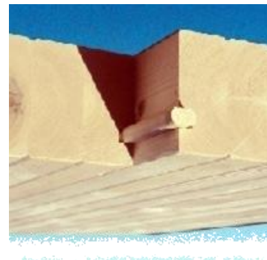
Figure 4.19, Wood pins to form a wall or floor, sources: Inholz.de , www.kaufmann-holzbau.de
