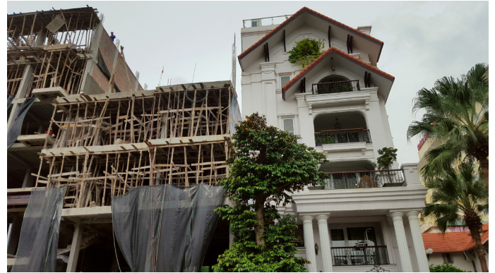
Image B.2.4: Construction work in Hanoi
