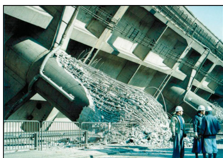
Fig. 2: An example of poor seismic design: the Hyogo-Ken Nanbu earthquake in Japan, 1995 42 (© Copyright 2018, Lecturas Digitales SA de CV)
