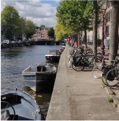
(a) Extensive horizontal displacement of the quay wall at the Prinsengracht
