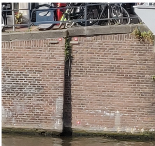
Figure 2.7: Installed SmartBricks around a displaced quay wall in Amsterdam
