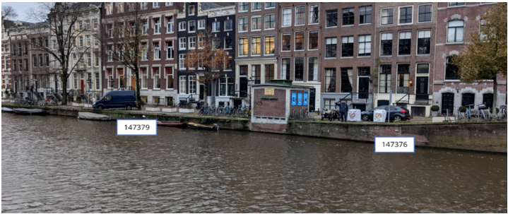
Figure 6.4: Location of the two SmartBricks placed on the SIN0401 quay wall
