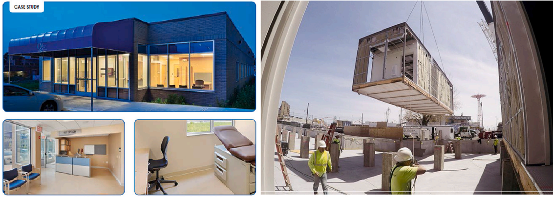
Fig. 22. Modular construction in hospitals example [66].
