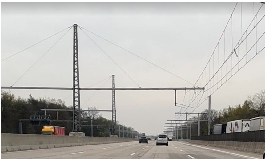
Figure 3.5: ERS construction located in the median of the highway (Google Maps n.d.)
