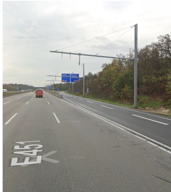
Figure 3.3: ERS construction located at an off-ramp (Google Maps n.d.)
