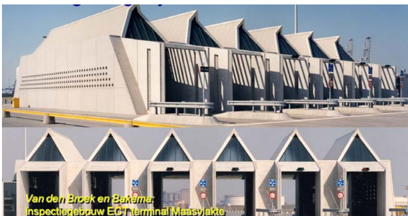
Figure 3.6: Application of the principles of natural ventilation in the ECT terminal in Rotterdam
