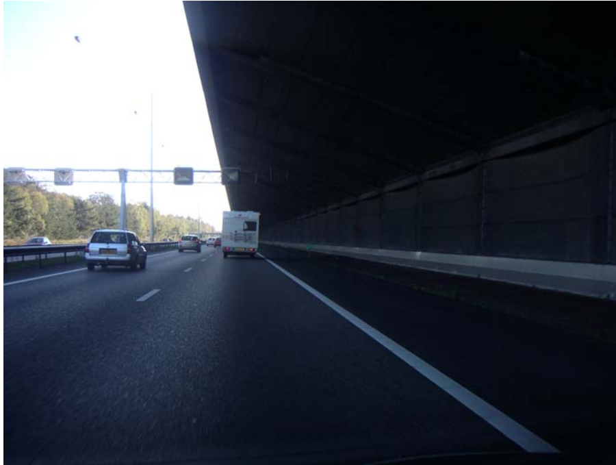
Figure 10. Extreme noise barrier (Zeist).
