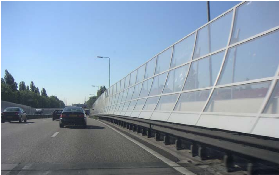
Figure 8. Effective noise reduction requires high, uninterrupted noise barriers (Rotterdam).
