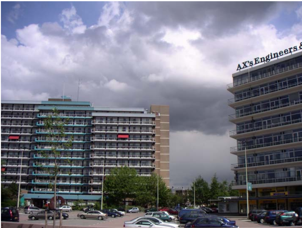
Figure 11. Non-continuous (detached) office buildings offer minor shielding.
