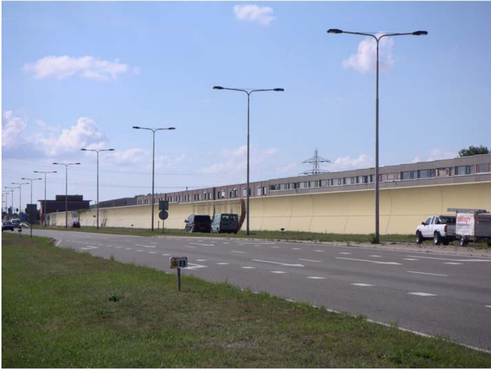
Figure 7. Noise barrier in Delft, curved to reduce reflections to opposite side.
