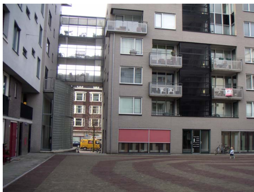
Figure 26. A passageway acts as a noise leak; hence as a secondary noise source.
