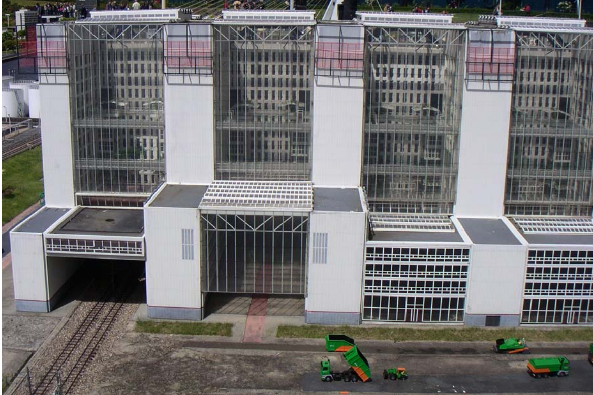
Figure 42. Office building with atria for noise control (Ministry in The Hague; scale model).
