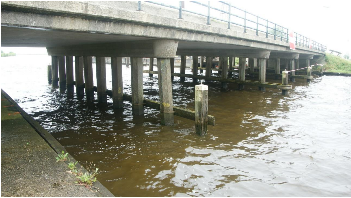
Figure 1. Photograph of Ruytenschildt bridge.
