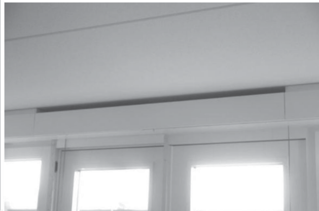
Figure 10. Example of air supply near the ceiling with the option of a curtain-location that will not disturb the air flow that enters the room (Renz Pijnenborgh).
