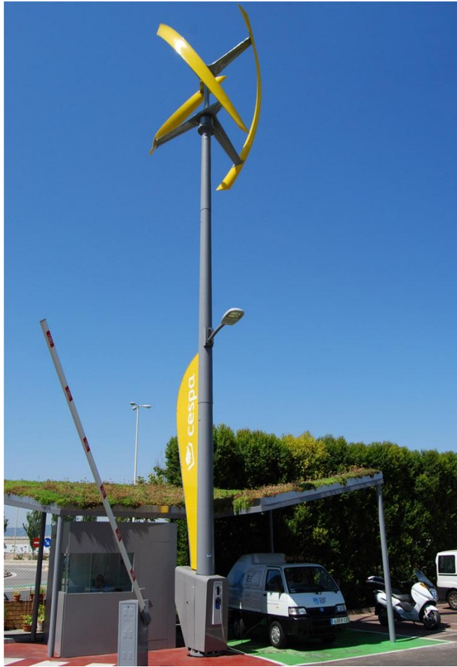
A Sanya Skypump EVCS installed in Barcelona, Spain. The system features General Electric's DuraStation charger and Urban Green Energy's UGE-4K VA wind turbine (UGE, 2012).
