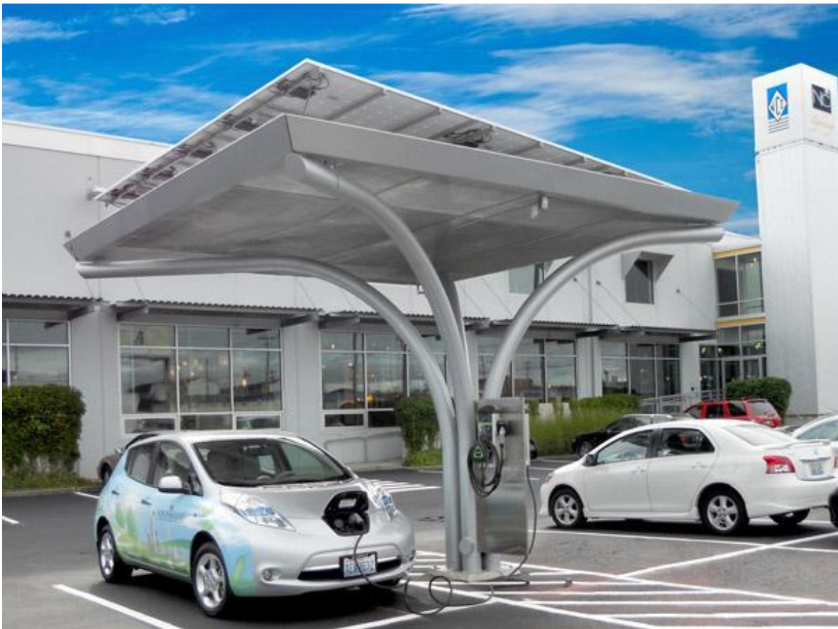
The 3.75kW Single Solar Canopy charging station installed in Seattle by EV4Oregon (EV4 Oregon LLC, 2011).
