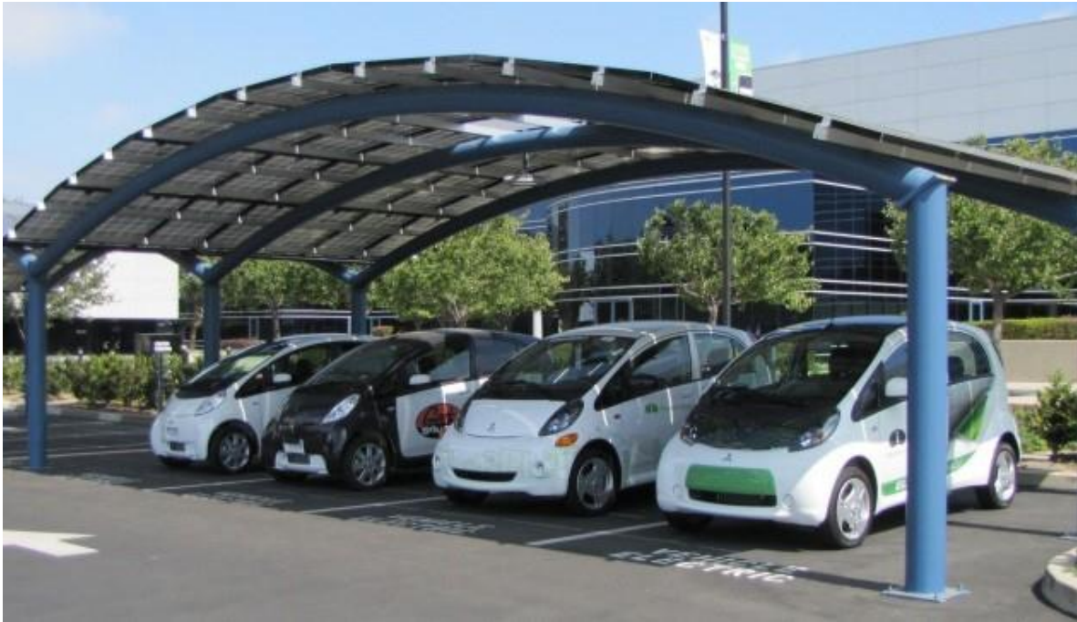
The 16.8 kW solar-powered charging station installed at the Mitsubishi Motors headquarters in Cypress, California (Mitsubishi Electric & Electronics USA, Inc., 2011).
