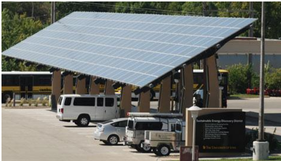
The 57 kW Solar powered EVCS in the University of Iowa (Facilities Management UIOWA, 2011).
