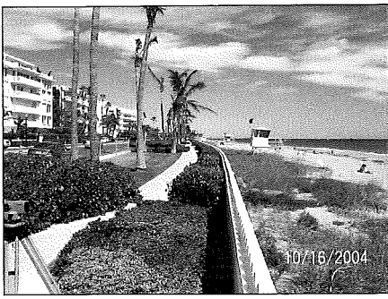
Figure 9. The Palm Beach Mid-Town nourishment project area soon after the passage of Hurricane Frances and Jeanne. The photograph was taken from FDEP monument R-98, view looking towards the north. The photograph was taken during the post-hurricane beach profile surveys (notice the survey level instrument on the lower left corner of the
