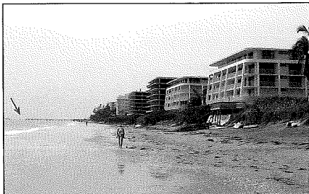
Figure 10. Non-nourished beach located less than five miles south of the Palm project. Notice the undermined structures on the right-hand side of the photograph and the destroyed fishing pier indicated by the black arrow.
