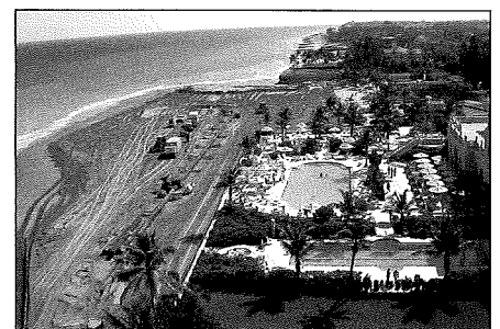
Figure 8. Construction of the Palm Beach 2003 beach nourishment project. The area illustrated is located south of The Breakers (between R-94 and R-95).
