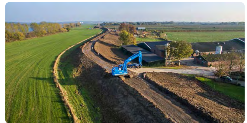
Figure 1: Construction of a dike. Source: HWBP (2018, p.103) , photo taken by Pascal Ogink.
