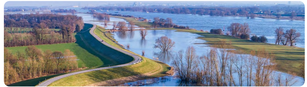
Location of a future dike reinforcement project along the river Waal. Photo via dijkversterkingwolferensprok.nl .
