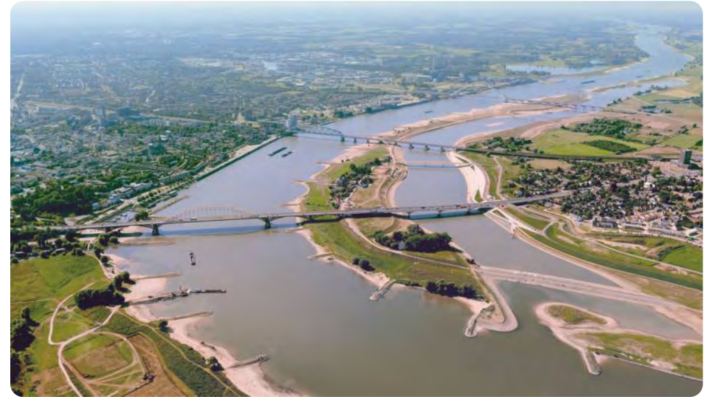
Current impression of the bypass near Nijmegen-Lent, with the old river dike still visible in between the two river branches. Photo by DaMatrix from Wikimedia Commons, CC BY-SA 4.0 .
