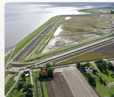
Double Dike. Photo by Waterschap Noorderzijlvest.
