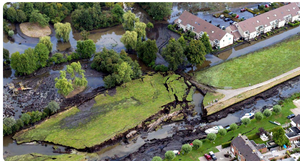
A sudden horizontal dike slide in August 2003 due to a hole of 60 metres in the dike flooded Wilnis. Photo © ANP.
