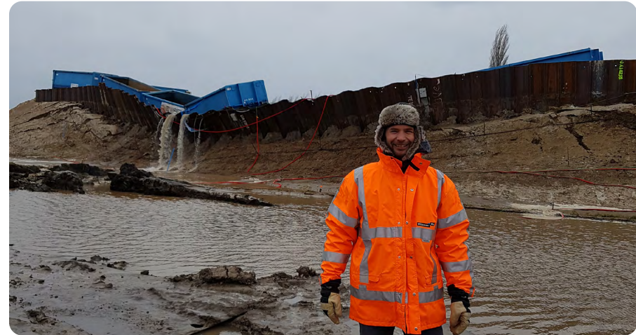
Figure 2: Eemdijk full-scale test; dike with sheet pile reinforcement after failure. Photo by Arny Lengkeek.
