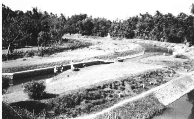
Figure 2 Vortex tube installed in canal in Java showing waste channel discharging into settling basin
