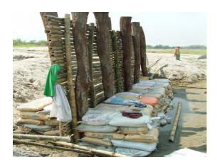
Figure 2.8: Vane pilot project, from (Douma and Mosselman, 2005).
