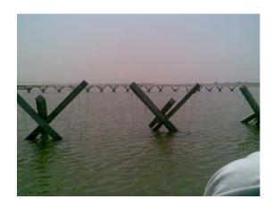
Figure 2.9: Jack Jetty screen for channel closure, from (Nayak et al., 2016).
