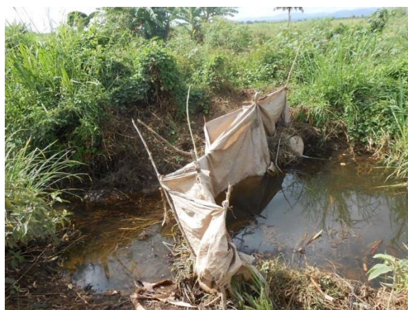
Figure 51: Blockage northern TPC drain near Kirungu
