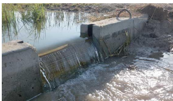
Figure 220: concrete weir with timber elements, side extension
