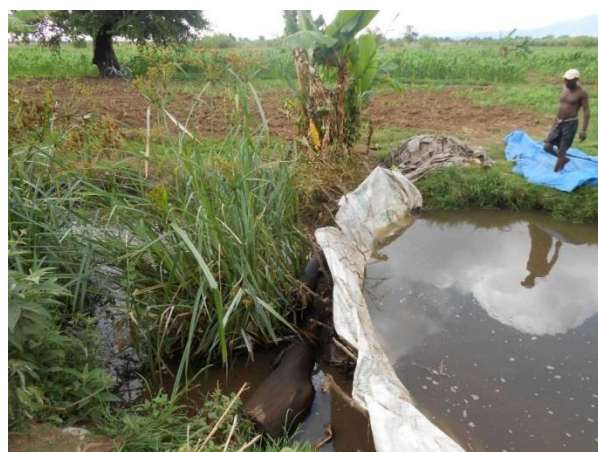
Figure 50: Blockage northern TPC drain near Samanga
