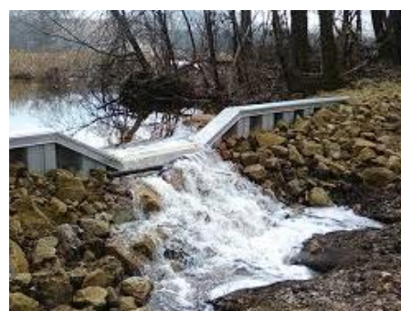
Figure 221: scouring protection with rocks
