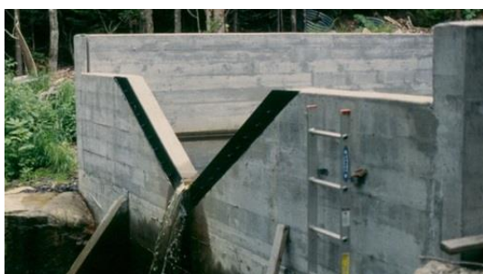
Figure 198: A V-Notch weir
