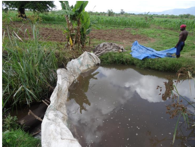
Figure 19: Blockage of TPC drain 1 near Samanga
