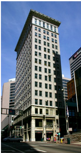
Figure 2.11: Ingalls Building in Cincinnati, US
