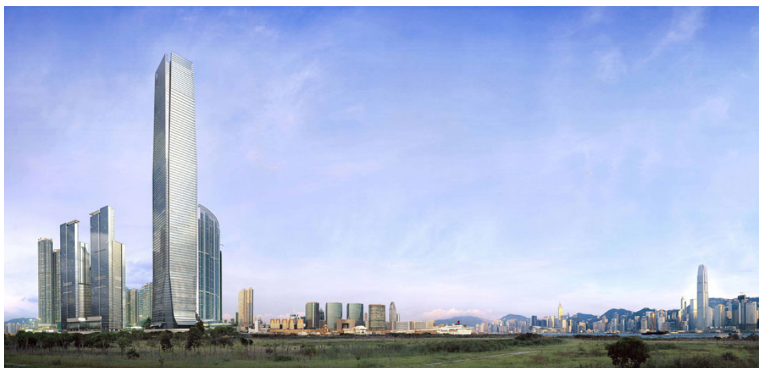
Figure 4.10: The International Commerce Centre, with on the background the Two International Finance Centre
