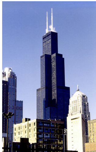
Figure 2.9: Sears Tower in Chicago, US
