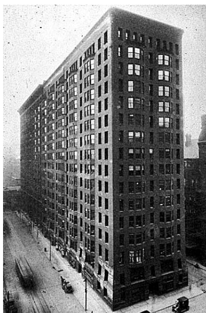
Figure 2.2: The Monadnock Building in Chicago, US
