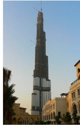
Figure 2.15: Burj Dubai under construction in Dubai, UAE
