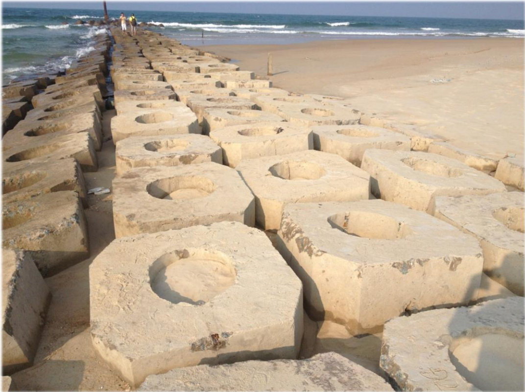
Figure 48: Sedimentated jetty on the most northwest part of the east-side of the barrier.
