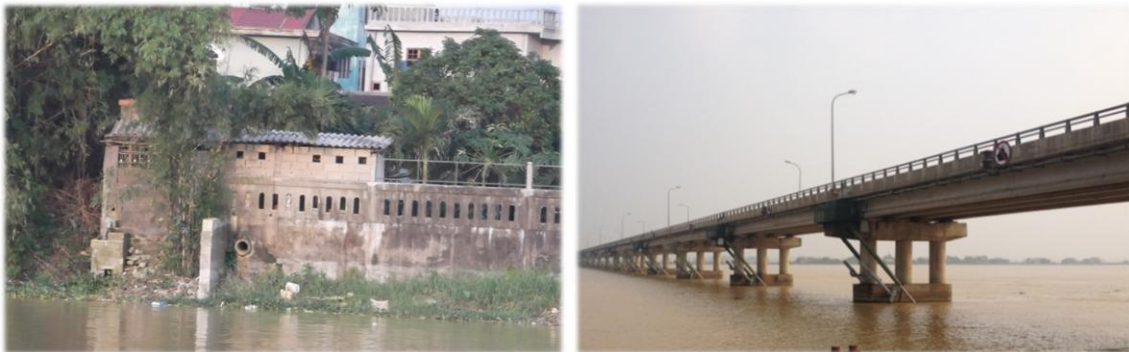
Figure 6: Sewage water running directly in the water (left) and the Thao Long dam against salt intrusion (right).
