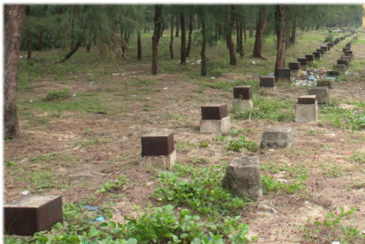
The pile row which was used as a start to close the Hoa Diem breach in 2000.
