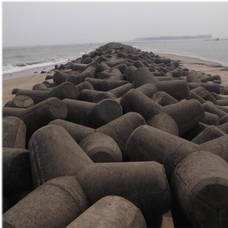
The north breakwater, build with Tetrapods, looking towards the lagoon.
