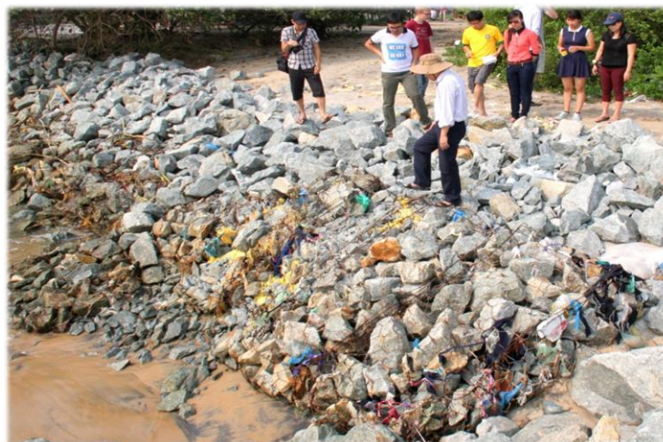
Grids on revetments capture a lot of litter... Maybe a solution?
