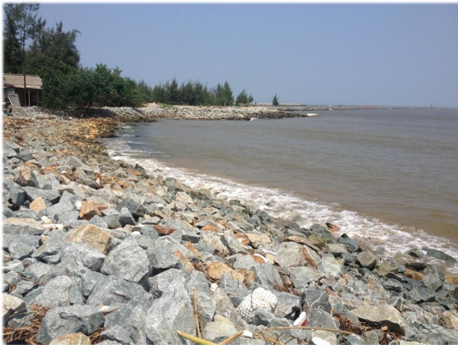
Figure 30: Working revetment on the east side of the west-barrier.
