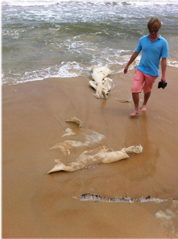
Figure 13: Leftovers of a geotube.
