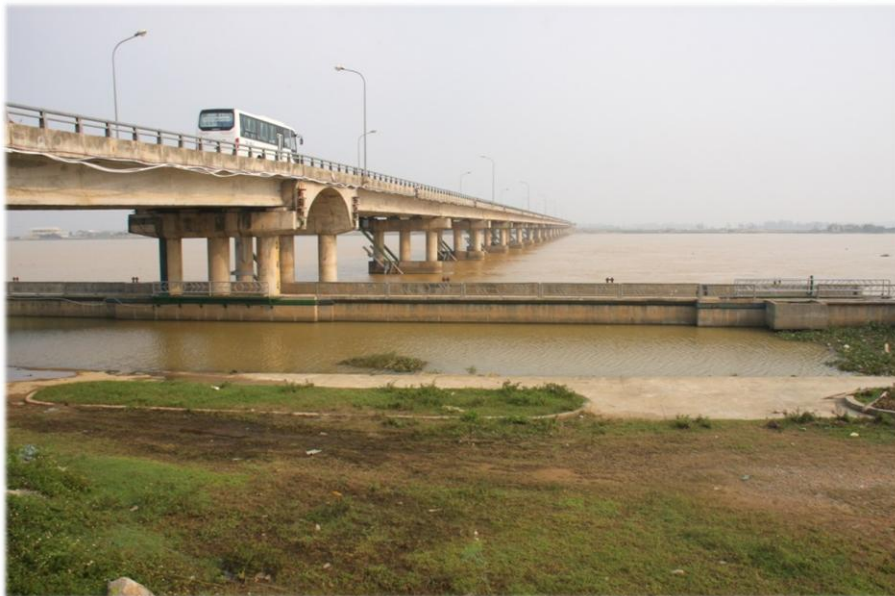
Figure 6: Thao Long dam, build to prevent salt intrusion. In front the ship lock can be seen, in the back the 15 gates with hydraulic arms.
