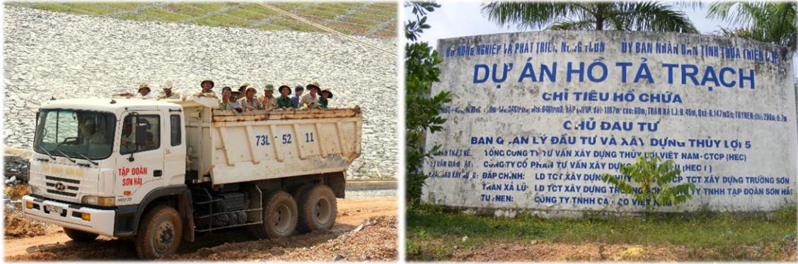
Figure 27: Workers at the Ta Trach dam (left) and information sign in front of the main office.
