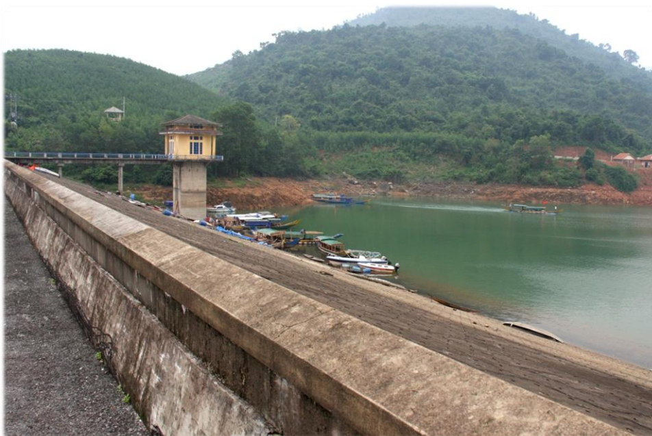
Figure 15: Maximum water level of the reservoir is indicated by the top of the red clay. The small wharf can be seen under the reservoir dam.
