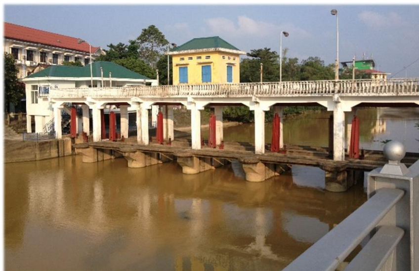
Figure 43: Phu Cam culvert
