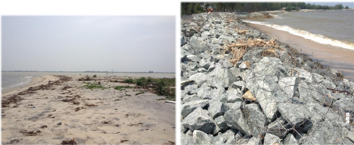
Figure 37: Sand spit growing (left) and the revetment (right) at the west-barrier.
