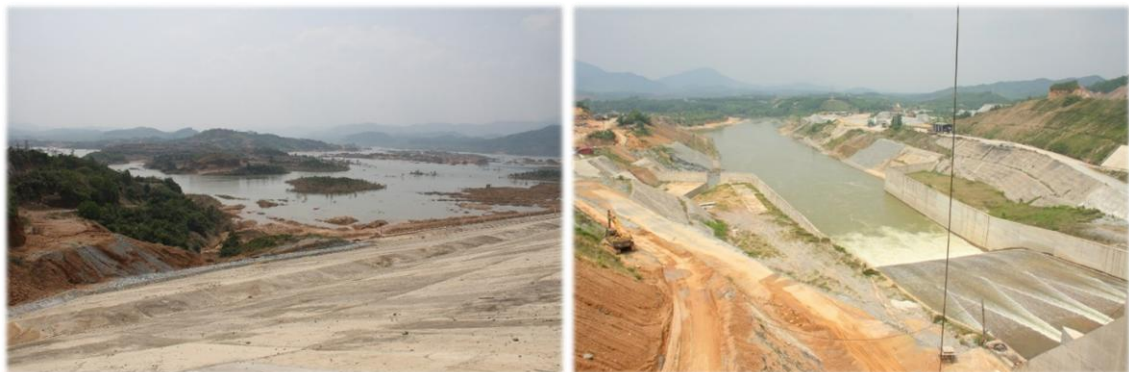
Figure 26: Ta Trach reservoir (left) and spillway (right)
