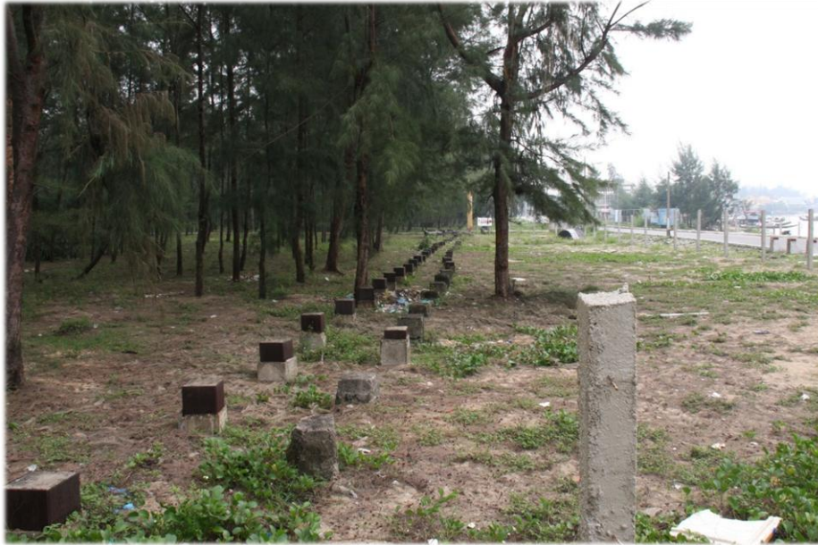
Figure 11: The pile row in the Hoa Duan inlet, which served as a basis for closing the breach.
