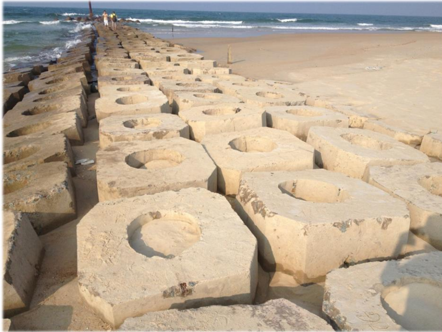
Figure 34: Sedimentated jetty on the most northwest part of the east-side of the barrier.
