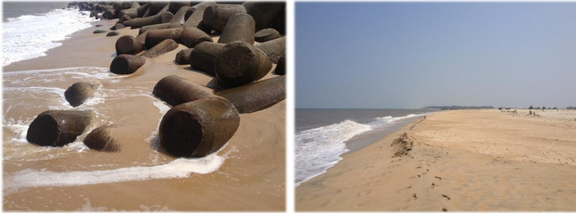
Figure 39: Sedimentated Tetrapods (left) and accretion (right).
