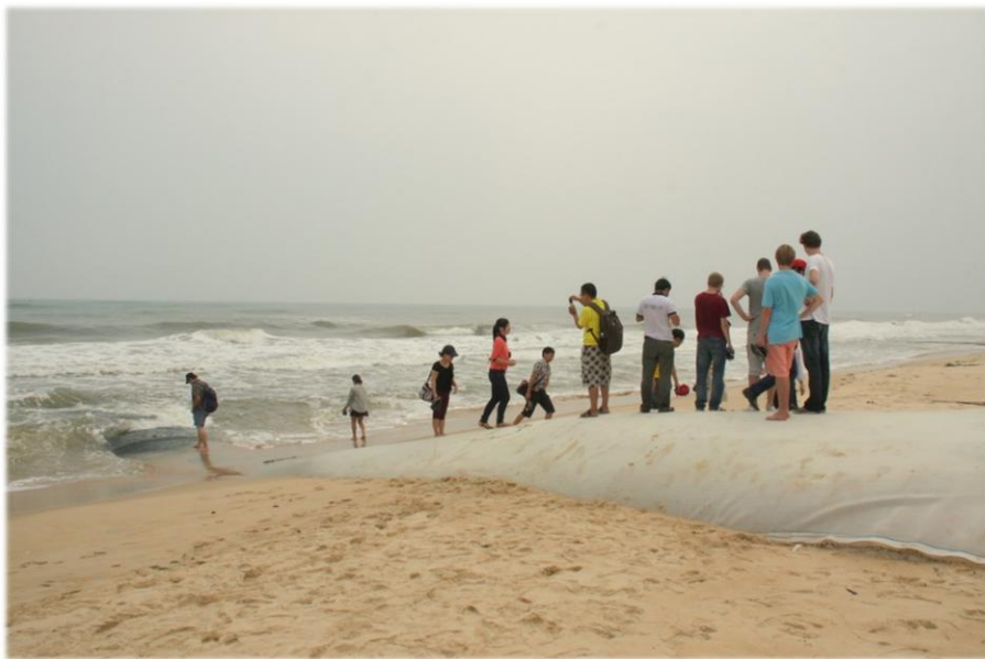
Figure 12: A deformed geotube, especially where the waves impact.
