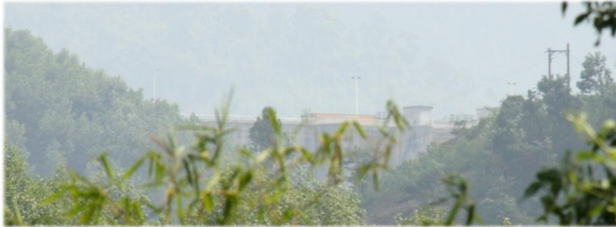
Figure 21: The Binh Dien dam from a distance.
