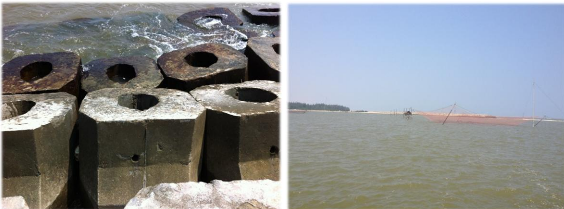
Figure 38: Failing modified Haros (left) and the basin with fishing activity (right).
