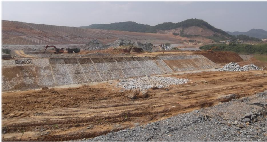
Figure 20: Ta Trach dam, with construction works in front of it.
