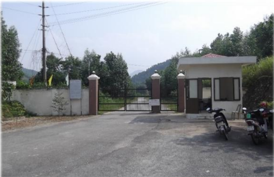
Figure 28: Closed gate at the Binh Dien dam.
