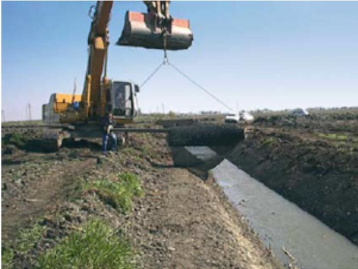
Figure 5. Installation of beaver netting along Zabarelle Canal
