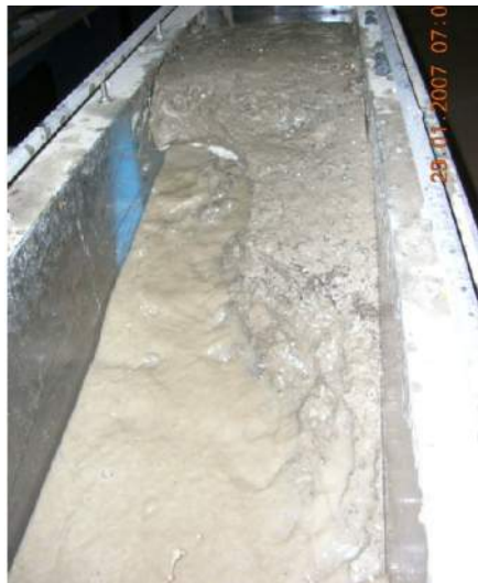
Figure 4-21 Damage did not start from the middle of the slope
