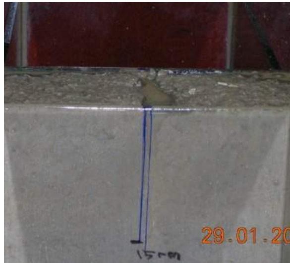
Figure 4-6 Damage at the surface after the sample hit by the impacts several times
