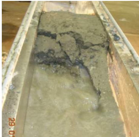
Figure 4-16 Fallen block of clay naturally protecting the slope from more damages for some time.
