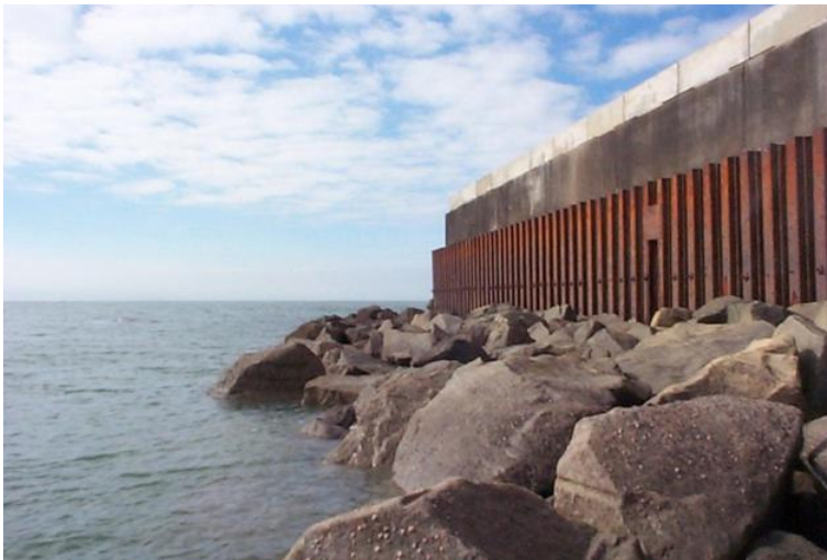
Figure 4.26 Samphire Hoe measurement site
